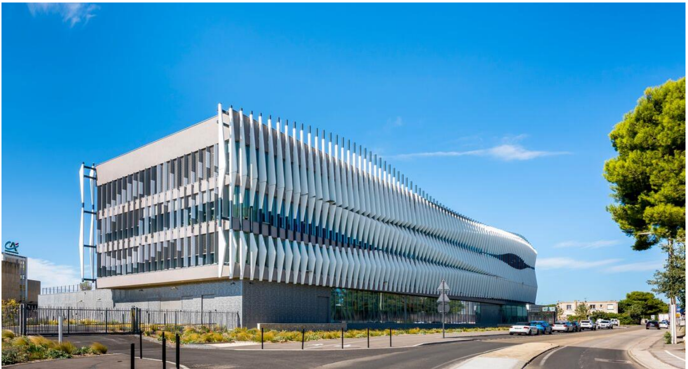
Crédit Agricole Building, Nîmes, France
