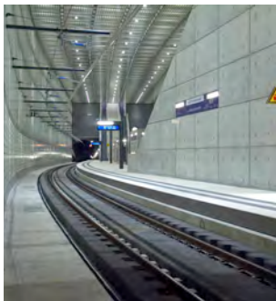
Leipzig City-Tunnel, Germany
