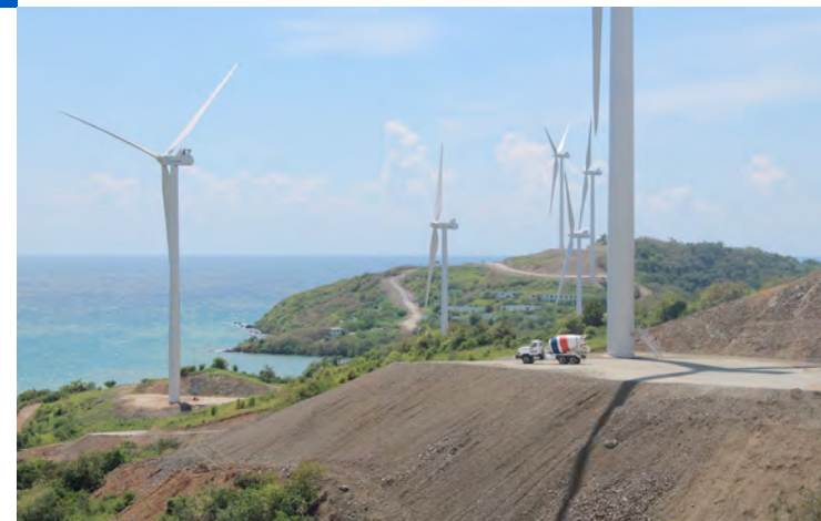
Wind Farm, Puerto Rico
